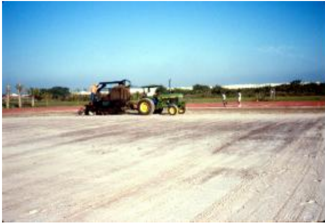
Birch matched renovation methods to field needs and budget resources. This field is sprigged rather than sodded.
